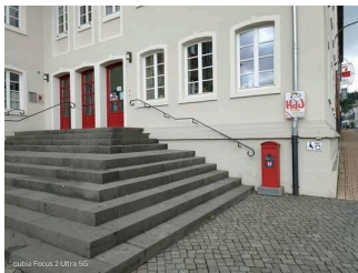
Main entrance (stair)
